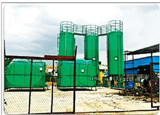
5 ton/day biogas plant at the Jawahar Nagar MSW dump yard in Hyderabad
