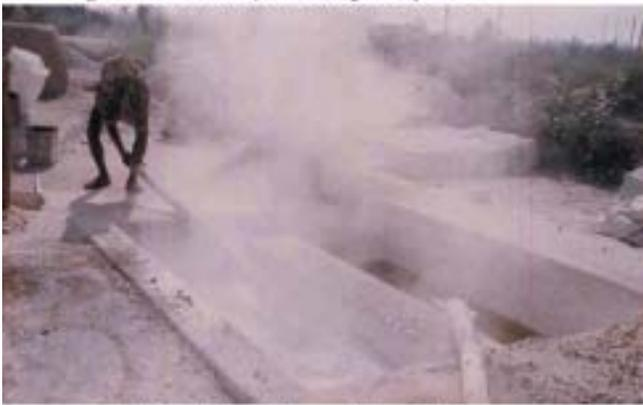
Fig.3 Stirring of lime during slaking
