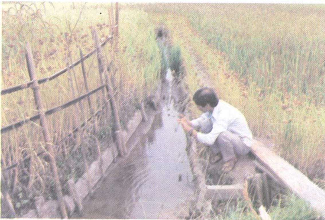
Fig. 3. Woon lining of primary irrigation channel in Apatani valley.
