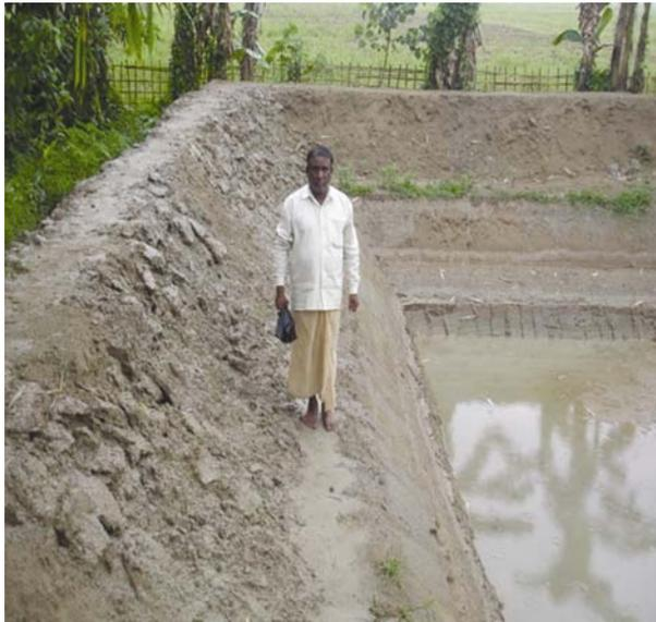
Fig. 3—Construction of tall and wide dyke for protection of pond from flood
