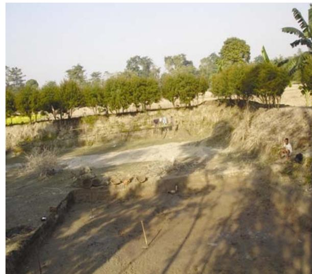
Fig. 4—Strengthening of pond dyke by turfing and plantation above the dyke
