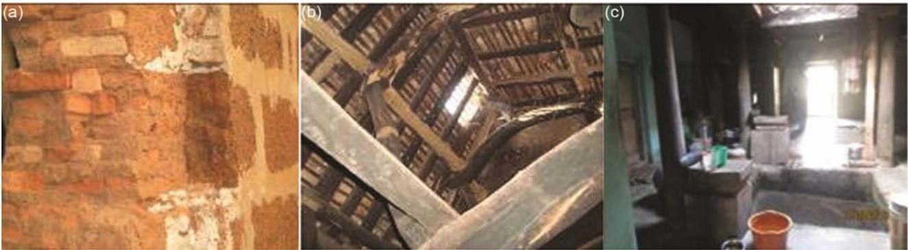
Fig. 6—Building components and construction techniques: (a) Flat brick wall with laterite block covering (b) Naturally processed wooden roof trusses (c) Courtyard at the centre aligned along the axis
